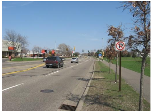
42nd Avenue N is a county road and a major thoroughfare in the city.
