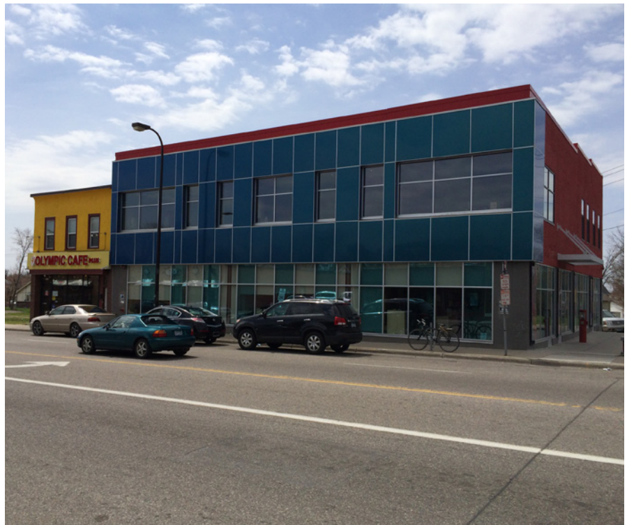
Building mass and scale intensifies at major intersections
