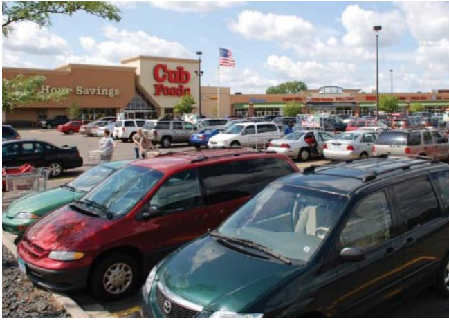
East side of Starlite Center strip mall
