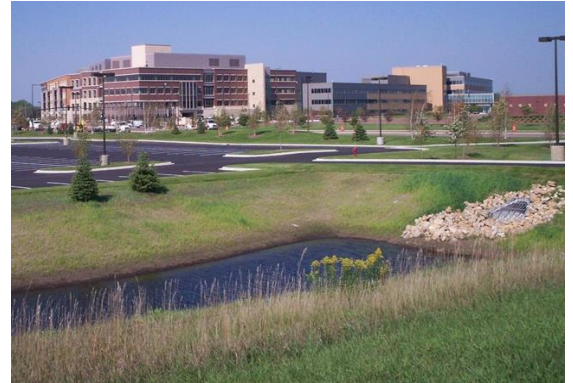
Target North Campus in Brooklyn Park, Photo from the City of Brooklyn Park
