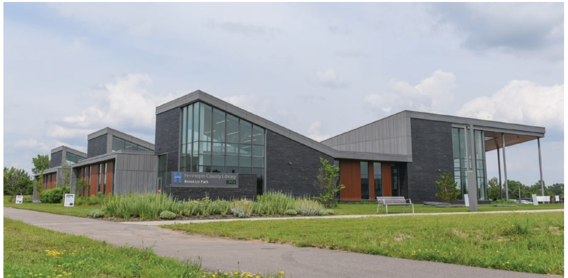
The Brooklyn Park Library adjacent to the 85th Ave LRT Station Area.
