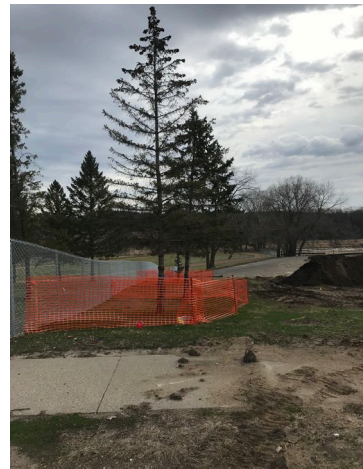
Tree protection at new Medical Examiners facility during construction
